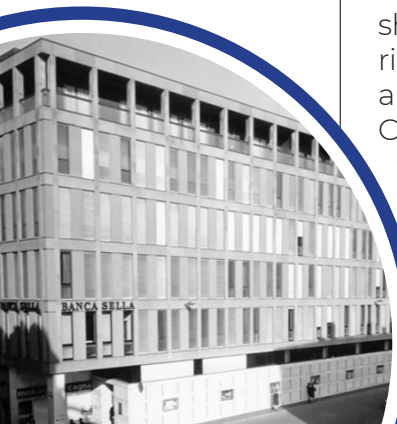
The building in via Italia, Banca Sella HQs since 1966
